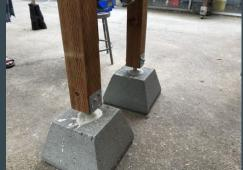
Pressure treated 4"x4" posts were fastened to cement pylons, creating the standing base for the bench
